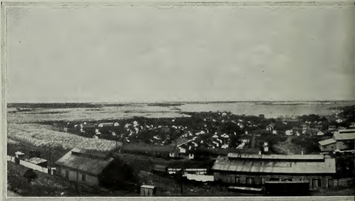
GENERAL VIEW OF PEARL
